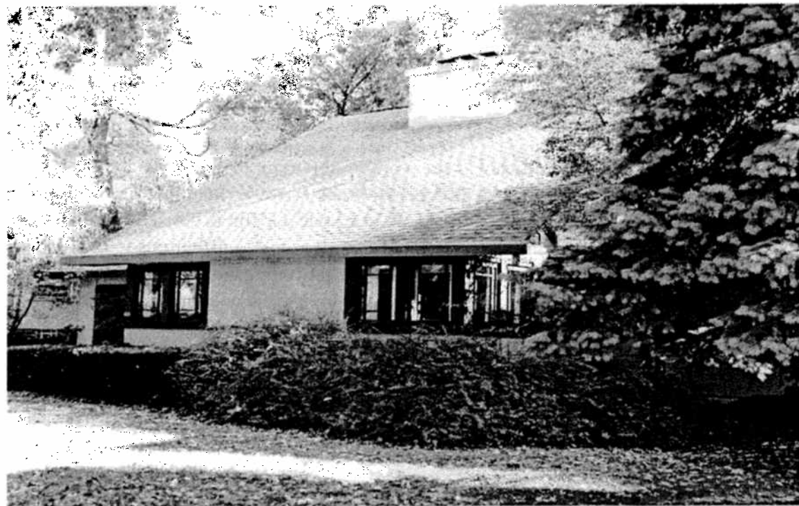
Top and above: The Peters House is a small, one-and-a-half-story stucco over frame building designed in the Prairie style.
